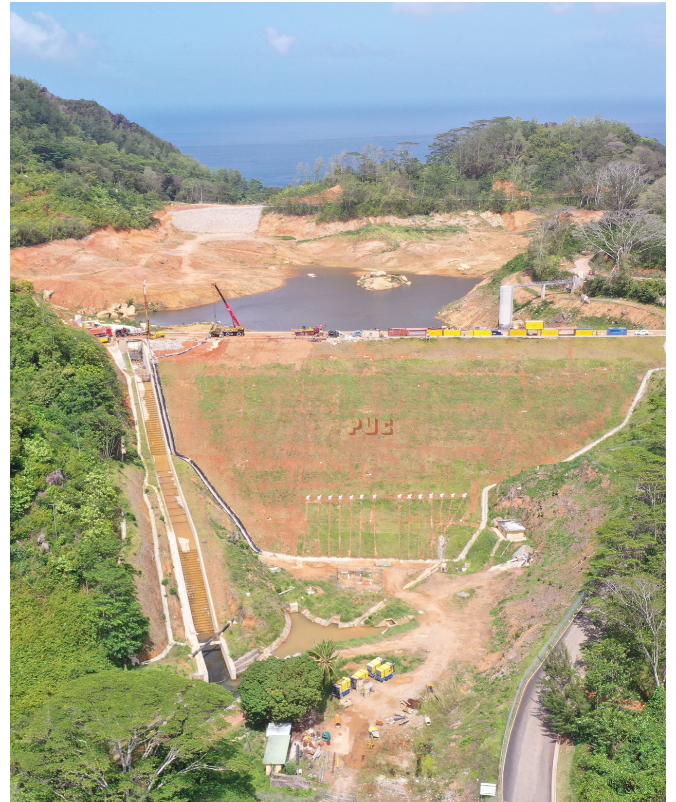
La Gogue dam - under construction. Source: PUC
